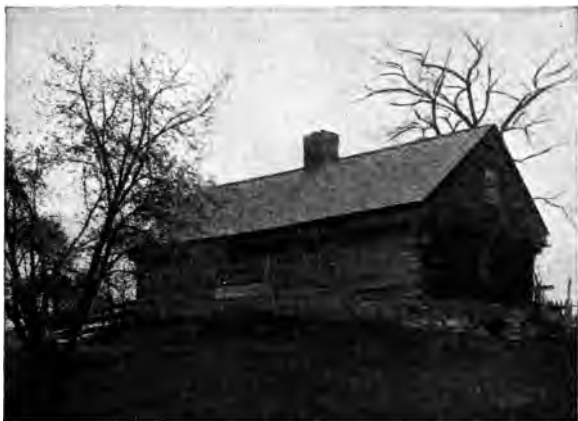
An old Dover garrison house that the Indians failed to destroy when they burned many neighboring buildings in 1688
